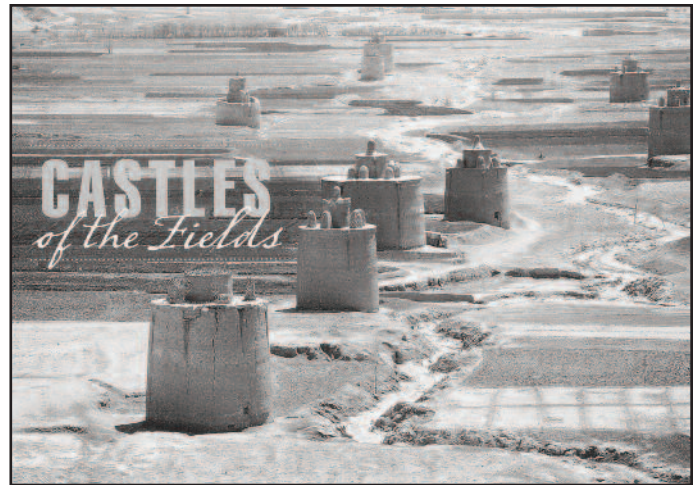
Though many of these towers look alike, no two are precisely the same.
